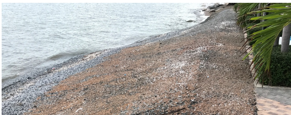
Figure 1 A polyurethane-bonded revetment in Thailand.
