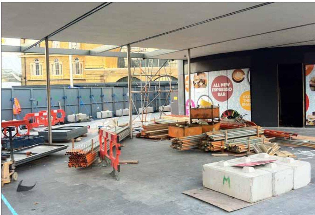
Figure 4. Construction in Granary Square (October 2013).
