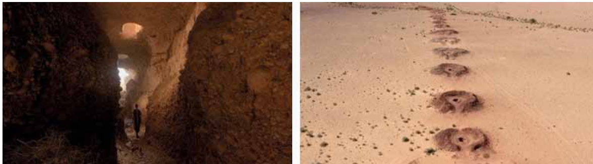
Figure 12. Khettara irrigation system in Figuig oasis, Morocco.
