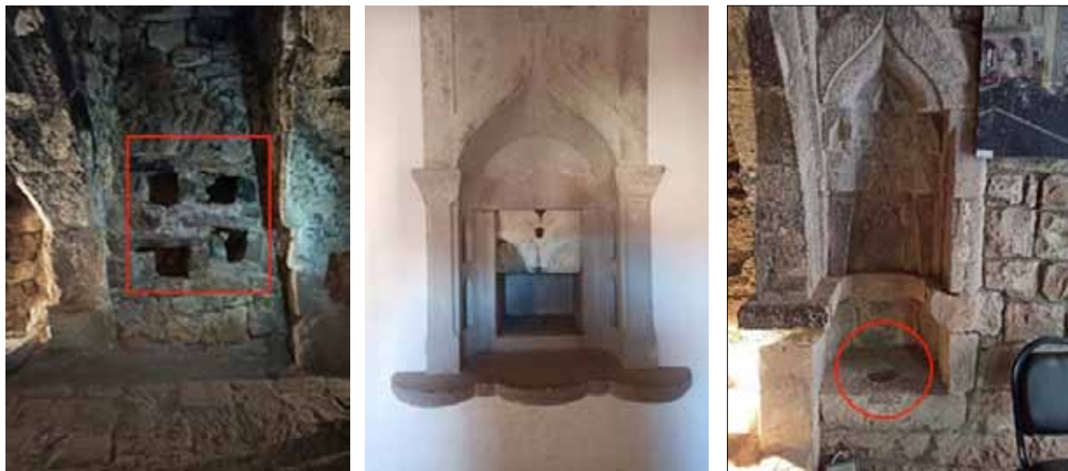
Figure 12. Left wall niches, called tembel delikleri and center & right serbetlik . (Source: Photo by authors).
