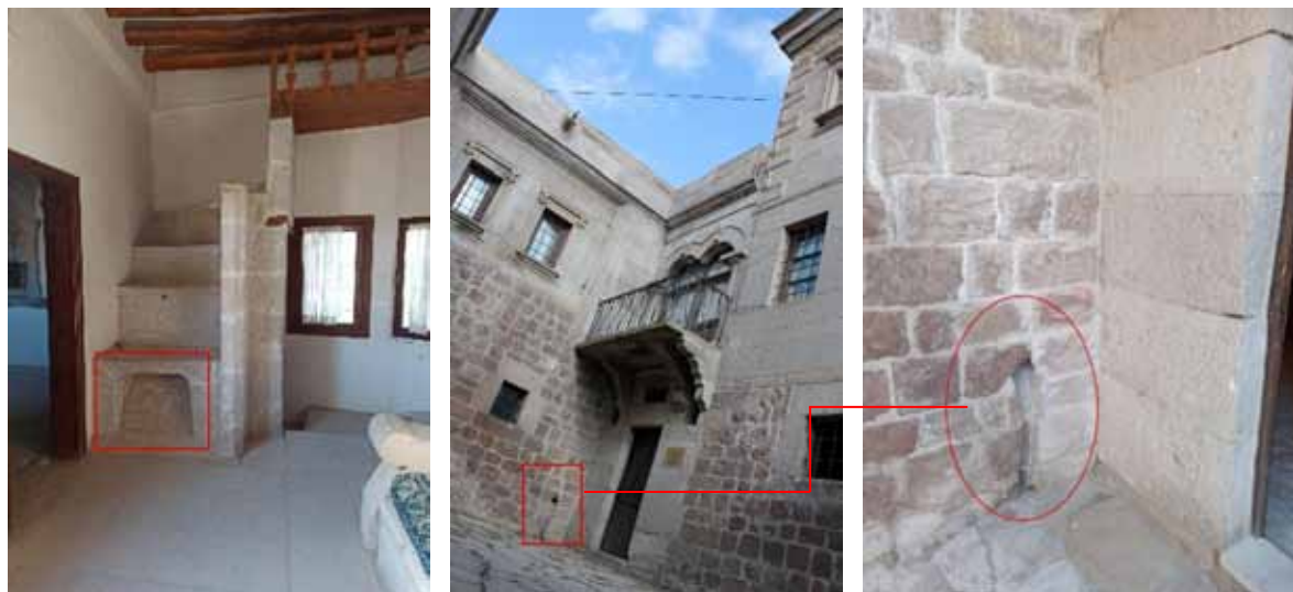
Figure 9. The staircase step also used as a sink and ablation space (a), and its drain in the wall (b-c) (Source: Photo by authors).
