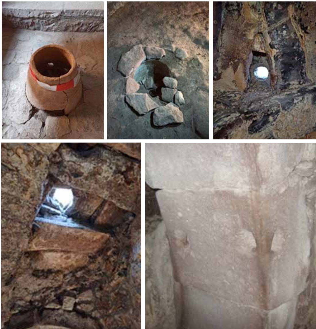
Figure 4. Views of the tandoor (top left) and the oven (top center) with their ventilation holes (top right & lower left) on the ceiling and stone arches with small holes for tethering the animals, in the carved rock-carved (lower right). (Source: Photo by authors).
