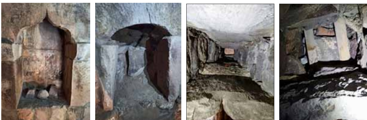
Figure 5. Built-in fireplaces (left) and interior views of their chimney extensions (right). (Source: Photos by authors).
