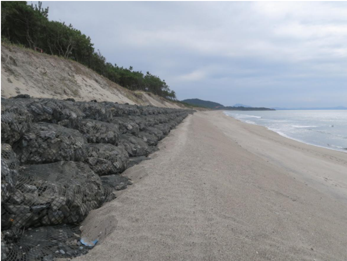
Figure 16 Close-up view of filter units taken at St. 6.
