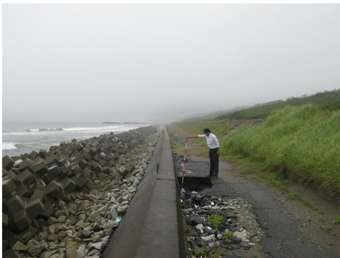
Figure 5 Artificial coastline protected by seawall and a number of concrete blocks.
