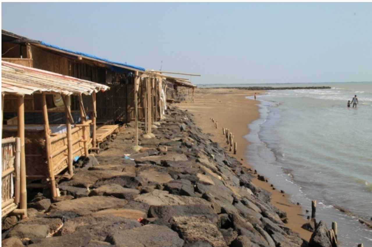
Figure 15 Sand deposits in front of CDS on east side of Truntum river mouth east jetty. Unregulated bamboo hut for tourism activity built on CDS. Photographed facing westward. Adopted from Setyawan et al. (2015).
