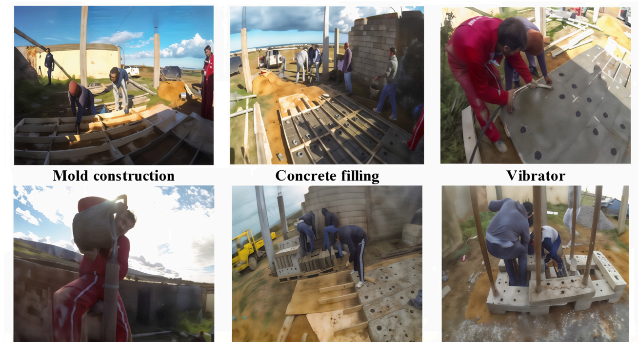
Figure 8 Stages of different modules construction of Oran reef 1 (O.R.1).
