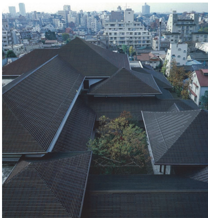
Fig. 7: Aerial view of the roof of the National Noh
