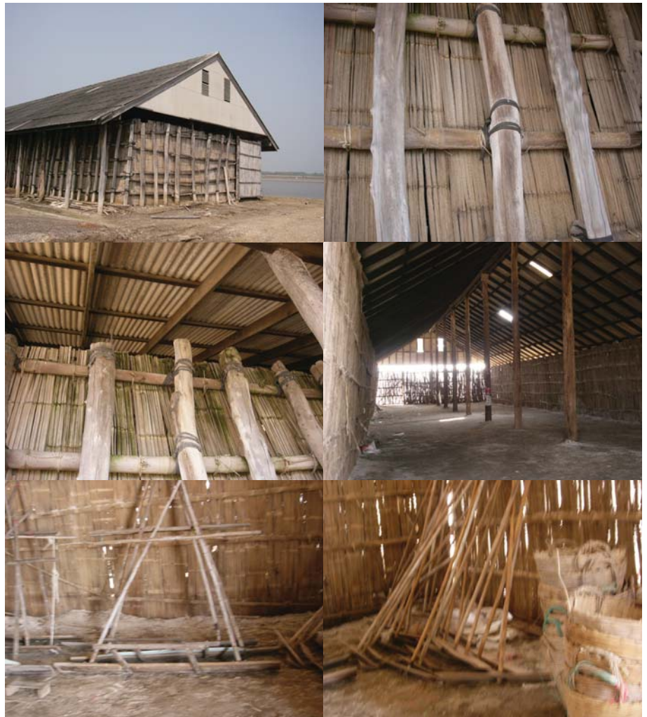
Figure 10 Salt barn and its details
