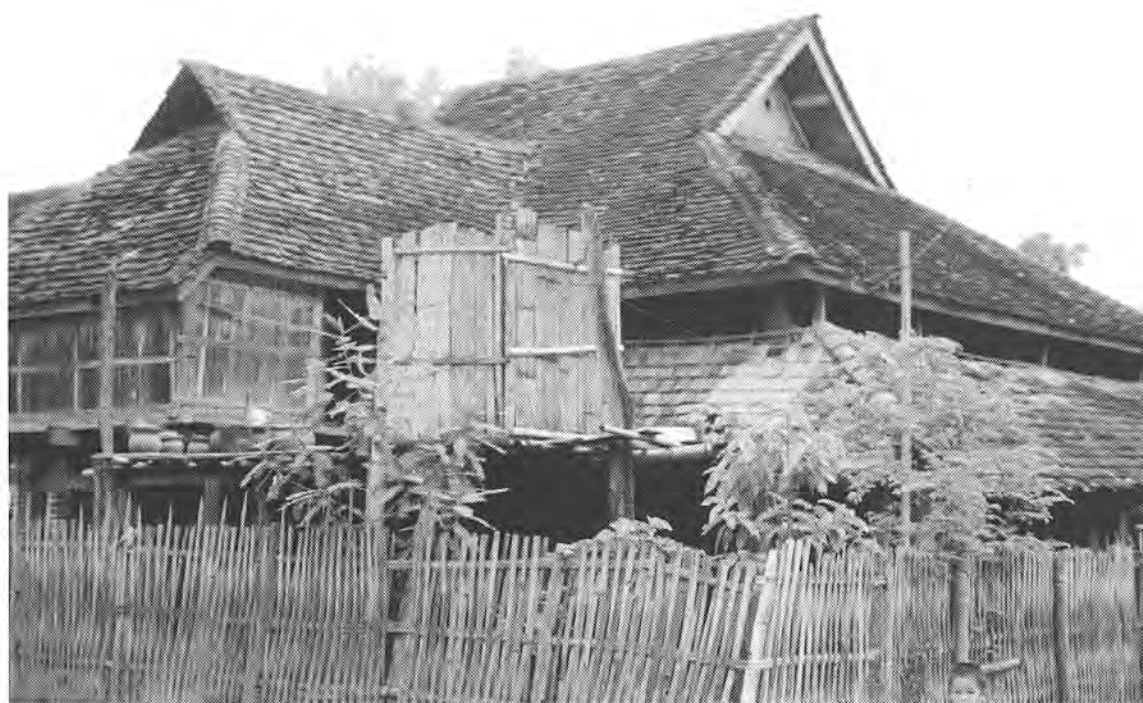
Figure 19 Roof form of Dai house in Sipsongpanna.
