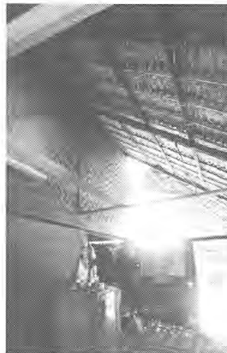
Roof's structure is built using bamboo and topped with Teak leaf.
