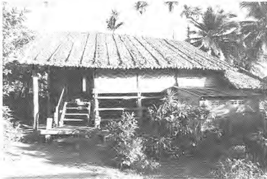
Entrance stair ladder
