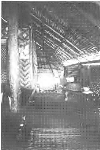
Roof's structure is built using bamboo and topped with Teak leaf.
