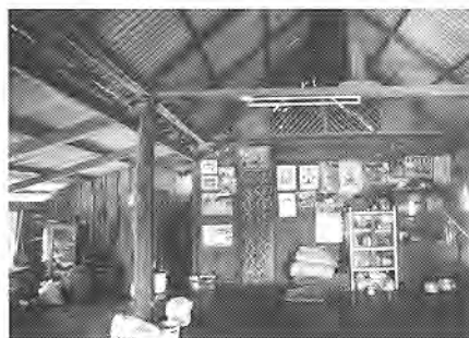
“Tern” and hallway to kitchen
