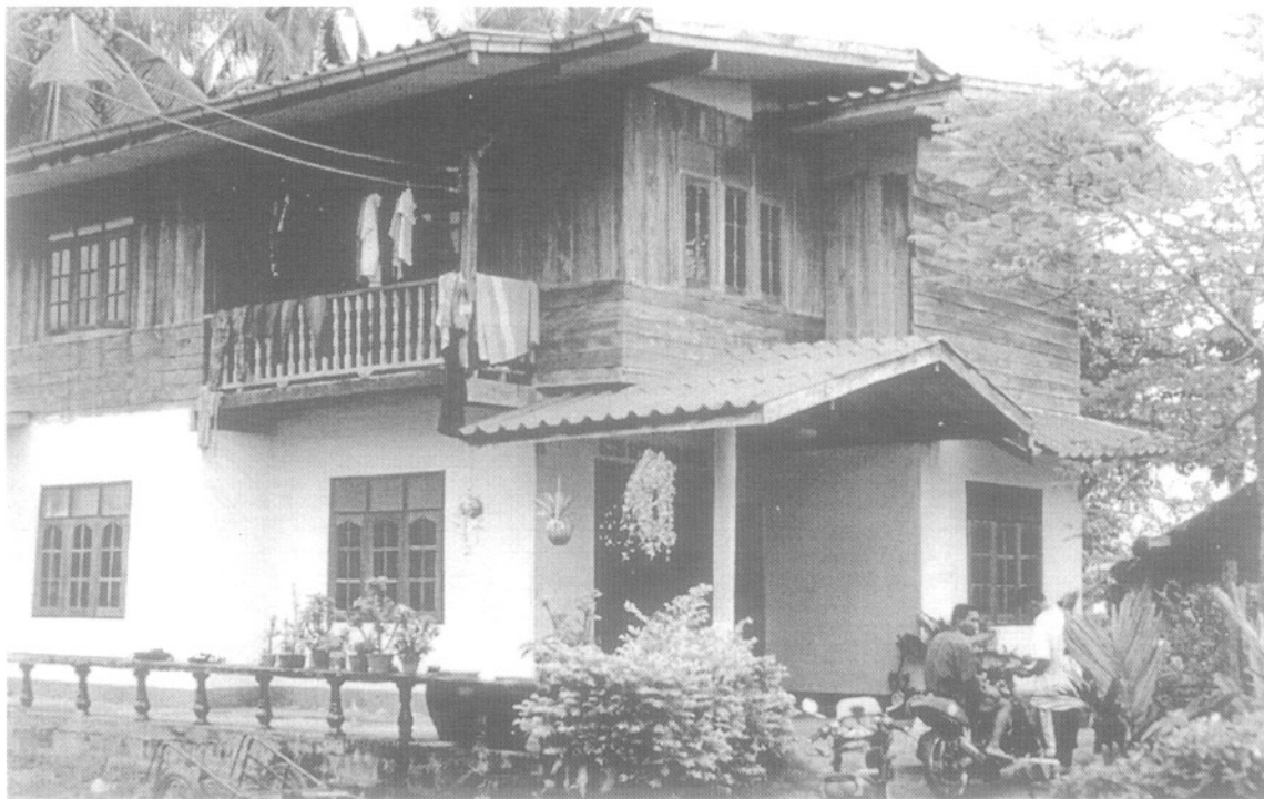
Figure 6 House # 3 Slightly modified house
