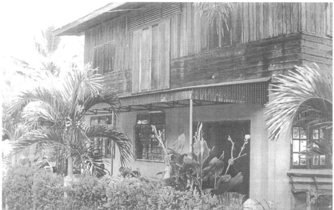
Figure 5 House # 2 Slightly modified house
