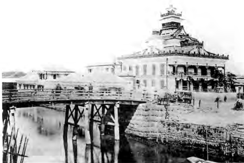
(5) Shimizu : First Mitsui Bank, Kaitunbashi, Tokyo, 1871-72. Unusual planning is seen at the double entrances and a strange location for the staircase.
