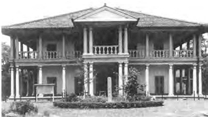
(3) Waters : Sempukan, the Mint at Osaka, 1868-71. The use of classical order and pedimental front with an open veranda plan.
