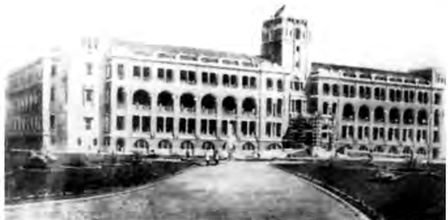
(32) Uheiji Nagano : Governor's Office, Taipei. Taiwan, 1910-1919. The twin quadrangle court plan proved to be practicable for Japanese public administrative buildings for some decades.
