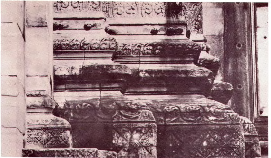
Figure 33. Southeastern rabbeted corner, base of Fig. 32. Shows good design and highly skilled craftsmanship.
