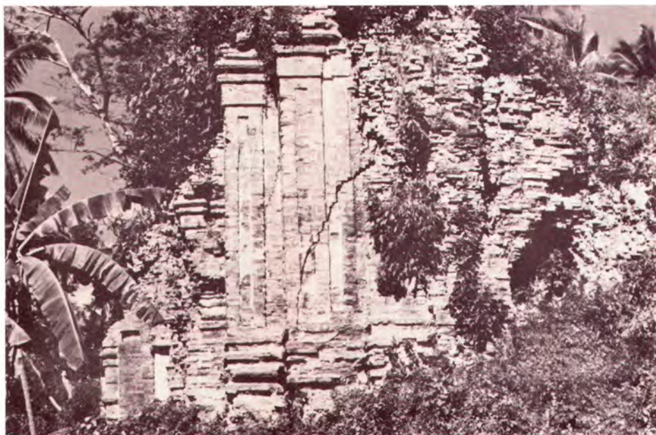
Figure 48. Chedi Wat Kaew, Chaiya District, Surat Thani Province. Peninsular Region/ Chaiya School. About 9th - 10th century A.D. The total structure was built with brick, then carved into various ornament patterns.
