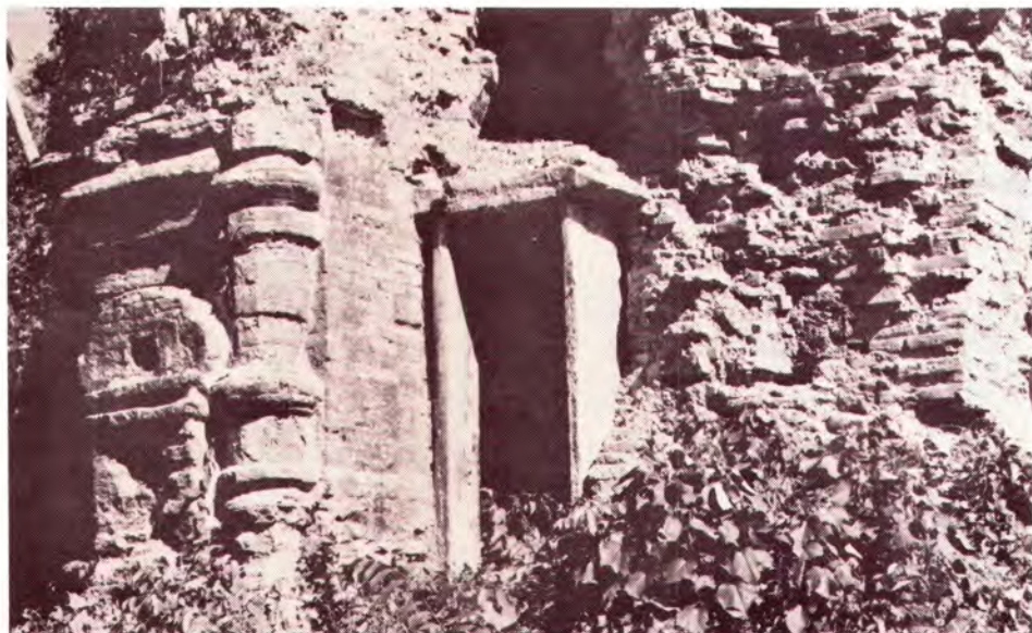
Figure 49. South elevation of Chedi Wat Kaew. Major architectural components were carved from its own brick structure, except the door frame of composite stone slabs.
