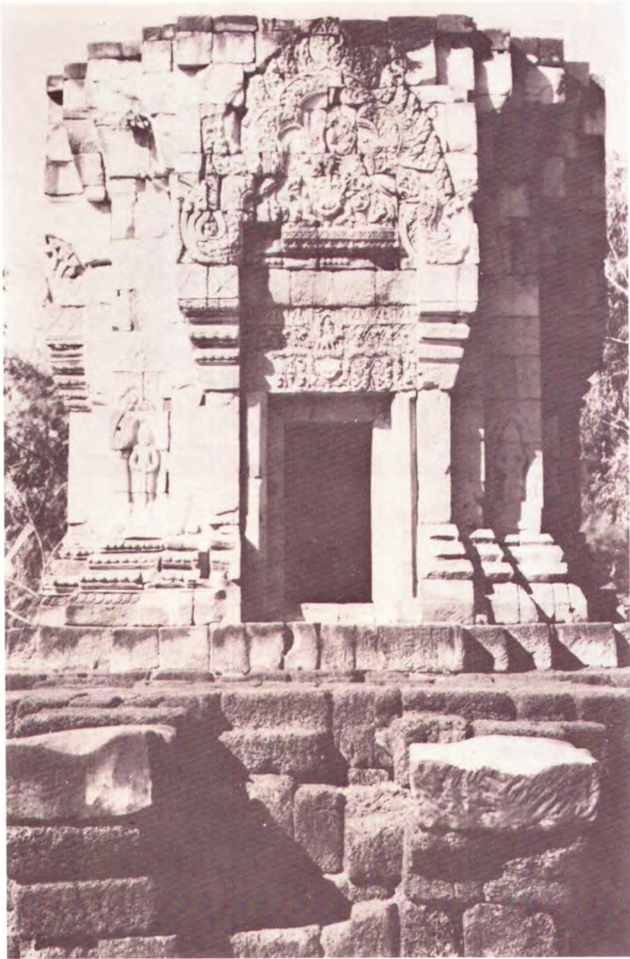
Figure 45. The main Prang of Prasat Ban Plueng, Surin Province. Later Part of 11th century A.D. The tower built with gray sandstone and the plinth with large laterite blocks.
