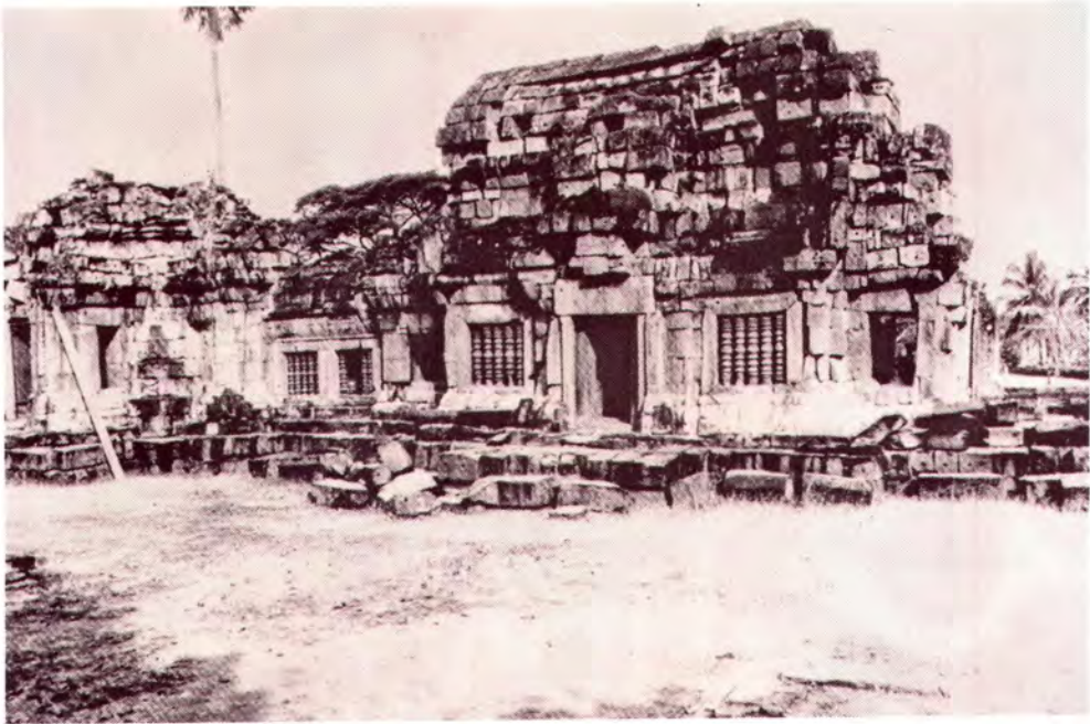
Figure 30. The main Prangs of Prasat Phanom Van, Nakhon Rachasima Province. Built with sand stone and unskilled craftsmanship, the super structure or tower had been demolished. Late 11th - early 12th century A.D.
