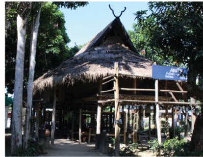
Demonstrated tortoise' shell-shaped circular Gables, Ban Na Pa Nad Tai Dam Cultural Center
