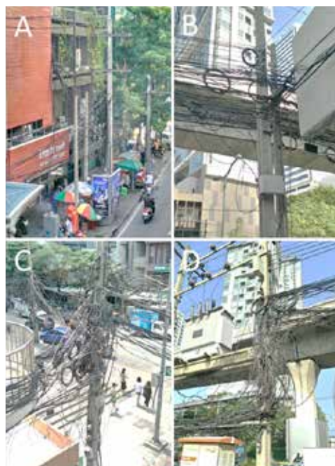
Figure 1. Typical view of a sidewalk in Thailand (A). The communication cable connected to the electrical power with hooks (B).The entanglement of communication cables (C).The communication cables/lines arrangement near the high voltage transformer (D).
