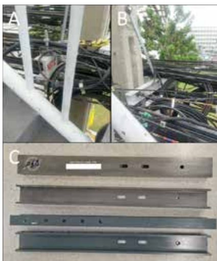
Figure 3. Installed FRP crossarm the front with NBTC logo (A) and the rear (B). FRP crossarm (glass fiber) supplied by Kij Sangthong Trading Co., LTD. (C)
