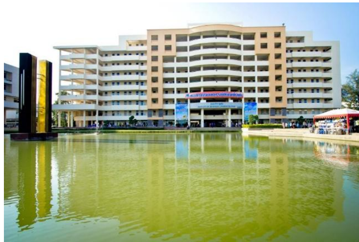
Figure 1 The existing exterior of the buildings of Faculty of Business Administration
