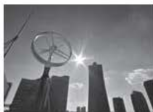
Compact wind power generator [MM Park Building]
