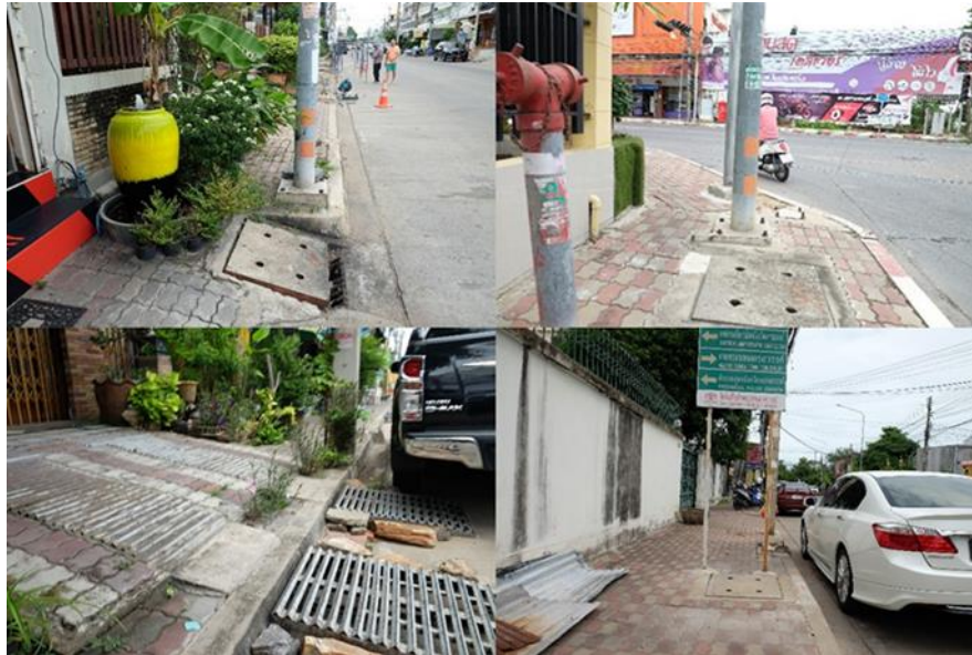
Figure 4 Examples of permanent obstacles on Vimarnman Road
