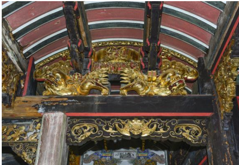
Figure 8 Gilded wood-carved beams of Jishan Lou building.
