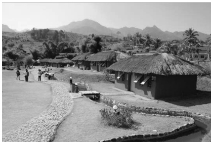
Figure 5: house built of clay soil mixed with straw or rice husks also known as Goo Fung
