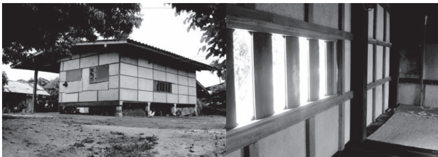
Figure 4, 5 Exterior and interior walls from natural fiber cement boards.
