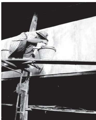
Figure 6 Repairing process from scrap of weeds to a new house.
