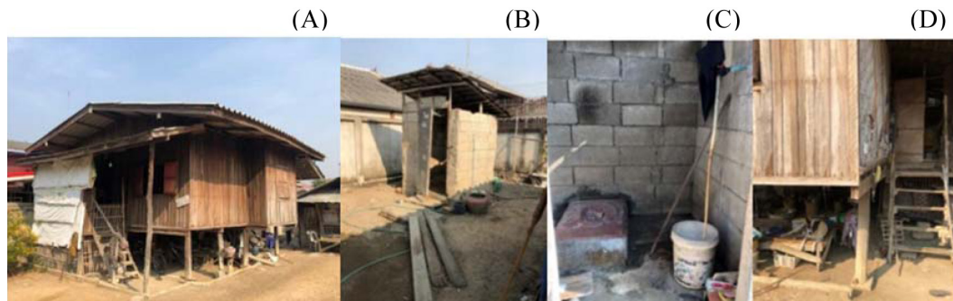
Figure 10 Bathroom outside the house in Chiang Mai before modification: (A) the targeted elderly house, (B) the bathroom without an appropriate pathway, (C) the squatter toilet, and (D) the steep ladder to the main living of elevated house
