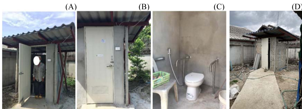
Figure 11 Bathroom outside the house in Chiang Mai after modification: (A) new bathroom with strong construction, (B) a column for roof structure, (C) seated toilet with handrails, and (D) an appropriate pathway to the bathroom
