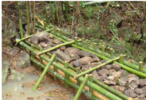
Figure 3 Rock-bamboo check dam
