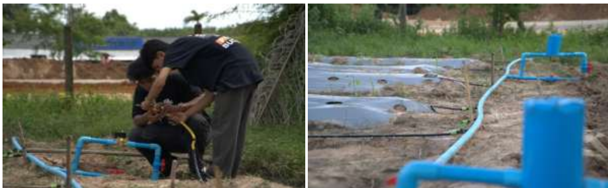
Figure 5: Installation of solenoid valves and connection of electrical wiring to the solenoid valves.
