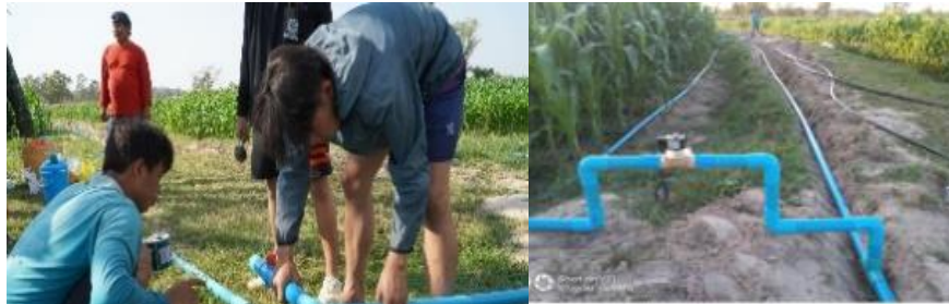
Figure 7: Laying out the water piping system along the crop rows.
