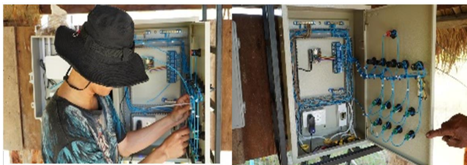
Figure 8: Developing and installing the control box
